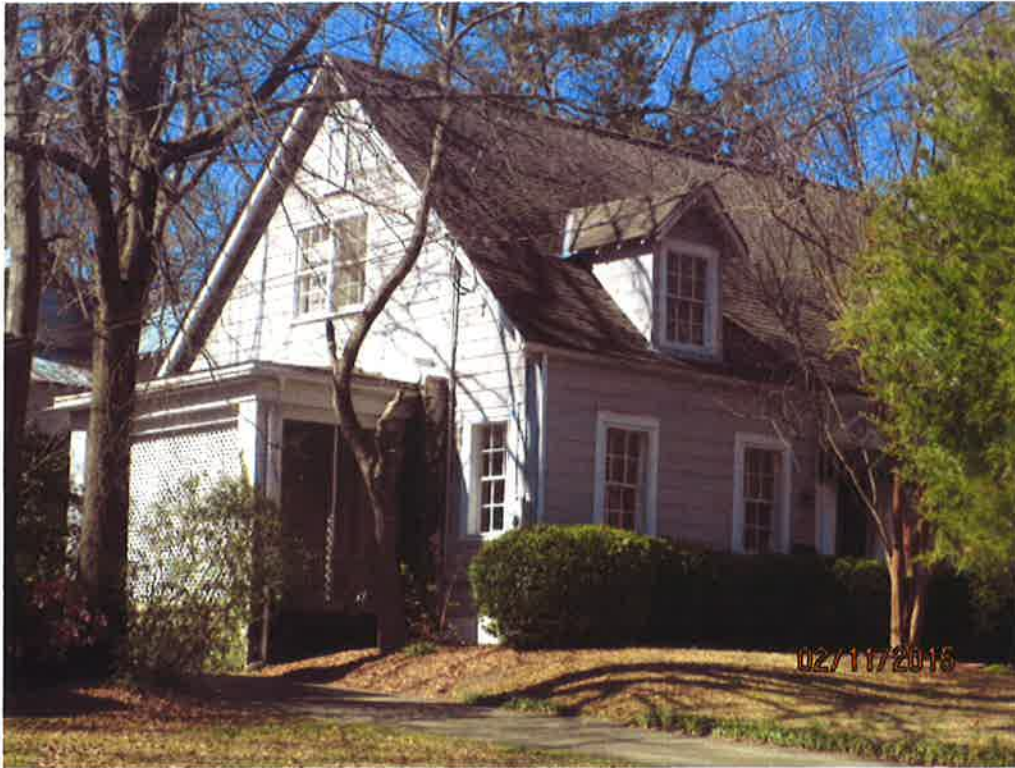
Partially removed chimney on College Street.
