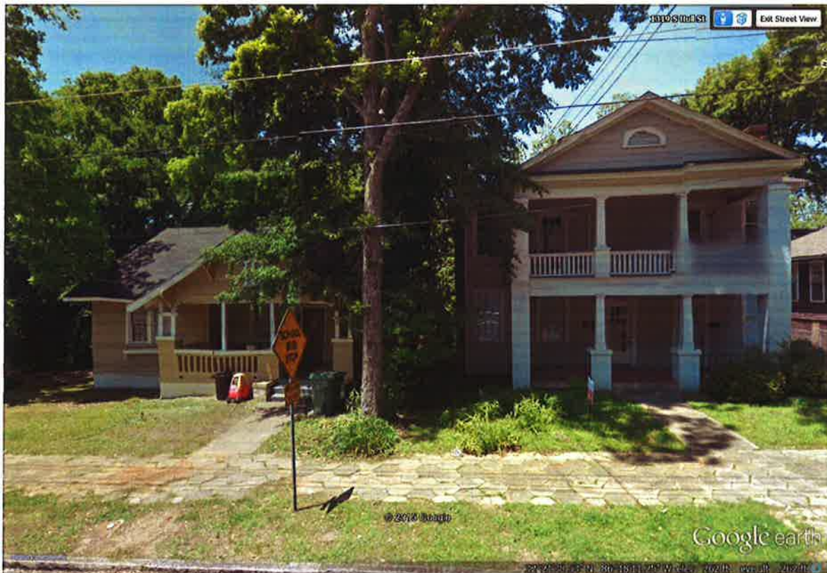
1314/1316 S. Hull Street
